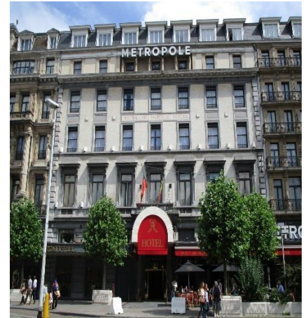
Metropolises in Brussels
